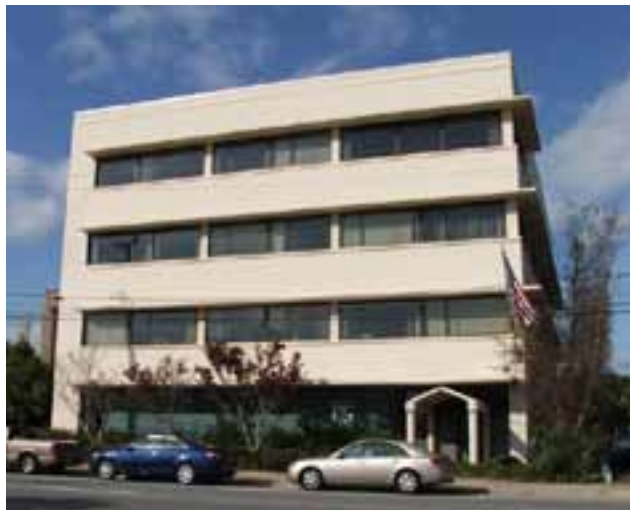
The 15,000-square-foot Center for Innovation and Entrepreneurship is located in Pensacola State College's downtown facility. The technology incubator is part of a multi-step strategy for developing critical entrepreneurial assets in Northwest Florida.
